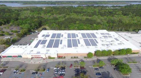
The 332.0kW DC roof mounted solar PV system was installed by Hannah Solar Government Services for the Target store in North Charleston, South Carolina. This system features Trina Solar 310W modules connected to Solectria 28kW inverters and supported by a Panel Claw mounting system. This system is part of the total 3 MW HSGS has completed for Target Stores across South Carolina.
