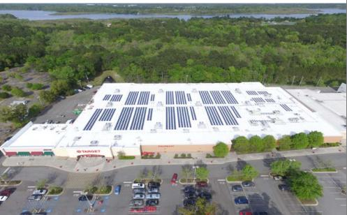
The 332.0kW DC roof mounted solar PV system was installed by Hannah Solar Government Services for the Target store in North Charleston, South Carolina. This system features Trina Solar 310W modules connected to Solectria 28kW inverters and supported by a Panel Claw mounting system. This system is part of the total 3 MW HSGS has completed for Target Stores across South Carolina.
