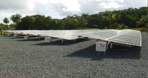
The 251.94 kW (DC) ground mounted solar PV system installed at the Ft. Buchanan Public Works Building in Puerto Rico provided by Hannah Solar Government Services features Suniva Optimus 255 Watt modules connected to a Satcon 250 kW inverter. The array is supported by a Solar FlexRack utility ground mounted system. Hannah Solar Government Services designed, engineered, and built the solar array. This renewable energy system will generate more than 359,172 kilowatt hours of energy annually.
