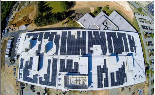
Hannah Solar Government Services (HSGS) was contracted by Gregory Electric Company to install a 1.35 MW ballasted solar PV system on the roof of the Trane Coil Plant located in Columbia, SC. Trane's solar array features 3,990 LONGI SOLAR modules, that are connected to 15 SUNGROW inverters and mounted by a Panel Claw racking system. The energy produced from this solar array will be used to assist in powering the Trane Coil Plant's day to day operations.
