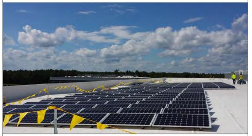
The 210.925 kW (DC) solar PV system installed on the roof of the New Jersey Army National Guard aircraft hangar in Lakehurst, NJ features a PanelClaw Polar Bear III ballasted mounting system on a flat roof. The system uses (2) AE 100TX inverters and SolarWorld's 275 watt monocrystalline solar modules. Hannah Solar Government Services designed, engineered, and built the solar array. This renewable energy system will generate 252,542 kilowatt hours of energy annually for the Department of Defense.
