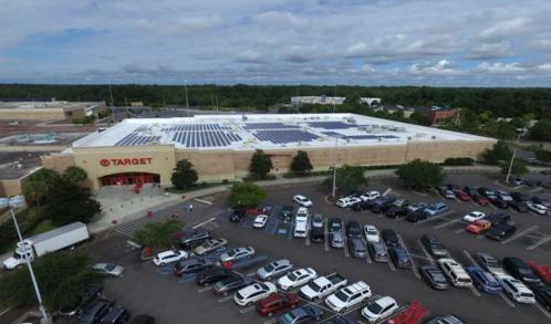
The 368.9 kW DC roof mounted solar PV system was installed by Hannah Solar Government Services for the Target store in Charleston, South Carolina. This system features Phonosolar 310W modules connected to Solectria 28kW inverters and supported by an Ecofoot mounting system. This system is part of the total 3 MW HSGS has completed for Target Stores across South Carolina.
