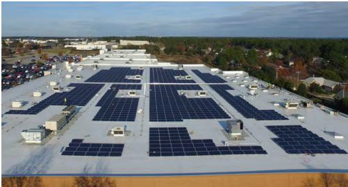
The 405.8kW roof mounted solar PV system was installed by Hannah Solar Governement Services for the Two Notch Road Target location in Columbia, South Carolina. It features Jinko 310W modules connected to (11) Solectria 28kW inverters. This array is supported by a Panel Claw mounting system. This system is one of 7 South Carolina Target stores that will be provided a total of 3MW of power.
