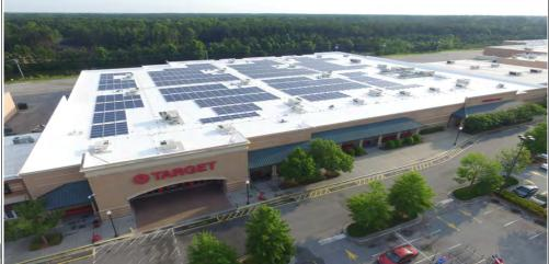
The 442.68 kW DC roof mounted solar PV system was installed by Hannah Solar Government Services for the Target store in Summerville, South Carolina. It features Phonosolar 310W modules connected to Solectria 28W inverters and supported by an Ecofoot mounting system. This system is part of the total 3 MW project for Target Stores across South Carolina.
