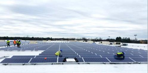
The 442.7kW DC roof mounted solar PV system was installed by Hannah Solar Government Services for the Target store in Aiken, South Carolina. This system features JA Solar 310W modules connected to Solectria 28kW inverters and supported by a Panel Claw mounting system. This system is part of the total 3 MW HSGS has completed for Target Stores across South Carolina.
