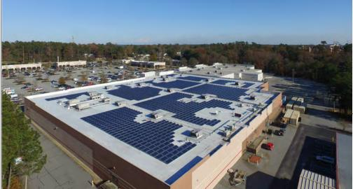
The 479.6kW roof mounted solar PV system was installed by Hannah Solar Governement Services for the Garners Ferry Target location in Columbia, South Carolina. It features Jinko 310W modules connected to (14) Solectria 28kW inverters. This array is supported by a Panel Claw mounting system. This system is one of 7 South Carolina Target stores that will be provided a total of 3MW of power.
