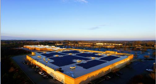
The 516.5kW roof mounted solar PV system was installed by Hannah Solar Government Services for the Target store in Lexington, South Carolina. It features Heliene 310W modules connected to (14) Solectria 28kW inverters. This array is supported by a Panel Claw mounting system. This system is one of 7 South Carolina Target stores that will be provided a total of 3MW of power. As of January 2016, this is the largest ballasted rooftop solar array constructed in South Carolina.
