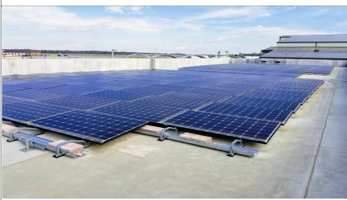
Hannah Solar Government Services (HSGS) was selected by Ahtna Technical Services Inc. to inspect and perform the preventative maintenance on a 27.5 kW DC solar PV system, fixated on the roof of the MCAS fitness center in Beaufort, SC. Services provided annually by HSGS for the maintenance of this solar PV system include: inspections of structural, mechanical, and electrical components, inverter testing, system voltage testing, grounding system tests, and module cleaning.
