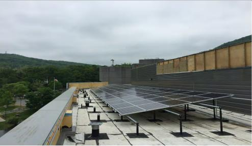
The 31.11 kW roof mounted solar PV system installed at the Keller Army Hospital in West Point, NY provided by Hannah Solar Government Services features Solar World 280 watt modules connected to 2 Advanced Energy 3-TL 20 kW inverters. The array is supported by a Silverback Solar roof mounted system. Hannah Solar Government Services designed, engineered, and built the solar array. This renewable energy system will generate more than 36, 490 kW hours annually.
