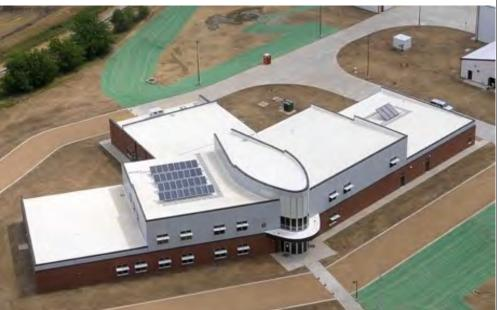
The 8.25 kW (DC) solar PV system installed on the roof of the new Army Reserve Center in Denton, TX features a Silverback Solar mounting system. The system uses a single 10 kW PowerOne inverters and Suniva's OPT250 250 watt mono-crystalline solar modules. Hannah Solar Government Services designed, engineered, and built the solar array. This renewable energy system will generate about 12,000 kilowatt hours of energy annually for the US Army.
