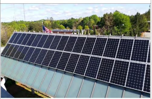
The HSGS team designed and installed the first solar photovoltaic (PV) system for a CDC facility. The system consists of 36 solar panels mounted to the roof using an Ironridge racking system. The array was custom designed to sit atop an existing walkway that leads to the entrance of the Visitor's Center and Museum. The solar PV system delivers 9.4 kW DC of clean power to the campus.
