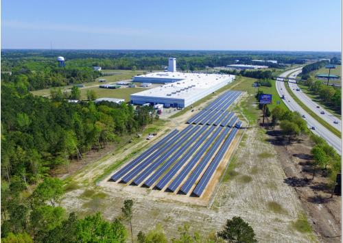
Hannah Solar Government Services (HSGS) designed, engineered, and installed a 1.22 MW ground mounted solar energy system for Otis Elevator located in Florence, SC. Otis' solar array features 3,660 Seraphim modules that are connected to SMA Sunny Tripower inverters and supported using a Solar FlexRack mounting system. In it's first year this solar array is expected to generate 1,852,700 kWh of energy which is enough electricity to power 171 homes.
