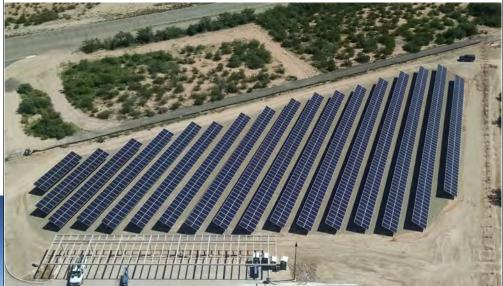
The 502.3 kW ground mounted solar PV system installed at Tucson International Airport in Tucson, AZ provided by Hannah Solar Government Services features SunPower 327W modules connected to (1) x 500 kW Solectria inverter. The array is supported by a RBI Solar ground mounted system. Hannah Solar Government Services designed, engineered, and built the solar array. This renewable energy system will generate more than 888,792 kilowatts hours of energy annually.
