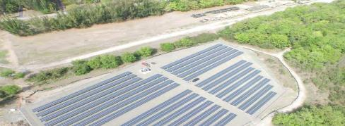
The 939.9 kW ground mounted solar PV system installed at the Ft. Allen in Juan Diaz, Puerto Rico provided by Hannah Solar Government Services features Sunvia 325W modules connected to a Solectria 500 & 250 kW inverter. The array is supported by a RBI Solar ground mounted system. Hannah Solar Government Services designed, engineered, and built the solar array.
