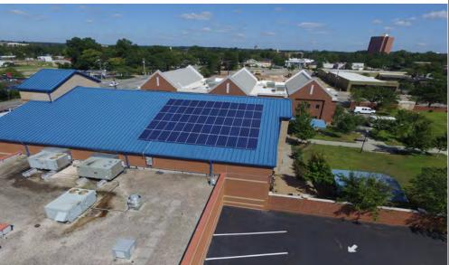
The 18.9kW DC metal roof mount solar PV system was installed by Hannah Solar Government Services for Midlands Housing Alliance in Columbia, South Carolina. This system features a Canadian Solar 315W modules connected to Solectria 14 kW inverters and supported by a Unirac roof mounting system.
