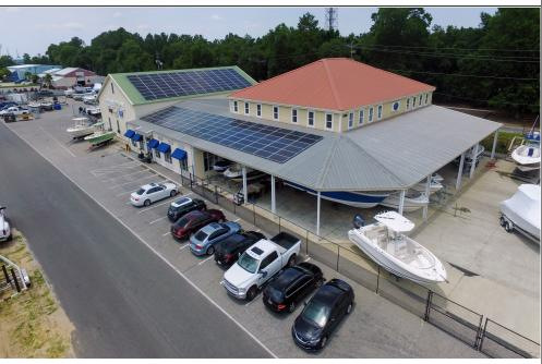
The 64.32 kW roof mounted solar PV system Hannah Solar Government Services (HSGS) installed on Longshore Boats features Canadian Solar modules connected to SolarEdge inverters and supported by Renusol MS racking system. HSGS designed, engineered, and built this solar array. Longshore's system is expected to generate more than 86,000 kW hours of electricity, annually.
