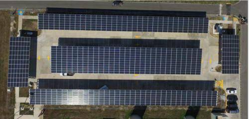
The 312kW solar PV parking canopy was installed by Hannah Solar Governement Services for Ft. Allen in Juan Diaz, Puerto Rico. It features Sunvia 325W modules connected to (1) Solectria 250 kW inverter. The array is supported by Schletter rails affixed to a Steel and Pipes canopy structure. Hannah Solar Government Services was responsible for the design, engineering, and construction of the solar array.
