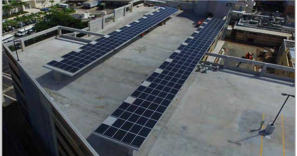
The 88.5kW solar PV parking canopy was installed by Hannah Solar Government Services for the Department of Veteran Affairs Medical Center in San Juan, Puerto Rico. It features SolarWorld 275W modules connected to (1) Solectria 75 kW inverter. The array is supported by Legrand Delta-strut rails affixed to the canopy structure. Hannah Solar Government Services was responsible for the design, engineering, and construction of the solar array.
