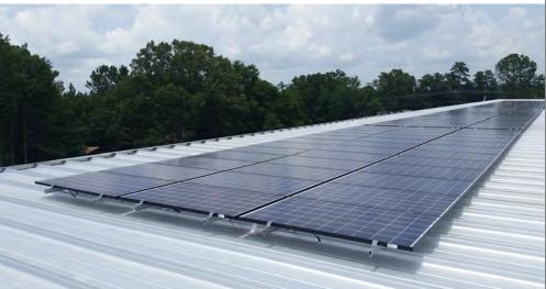
The 50 kW roof mounted solar PV system installed at Fogel Services in North Charleston, SC provided by Hannah Solar Government Services features (204) Trina Solar 250W modules connected to (3) x 14 kW Solectria inverters. The array is supported by a Unirac roof mounted sys-tem. Hannah Solar Government Services designed, engineered, and built the solar array. This renewable energy system will generate more than 57,820 kW hours annually.
