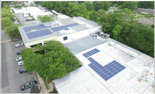
The HSGS team designed and installed two roof mounted solar PV systems for The GEL Group in Charleston, South Carolina. This system features Canadian Solar modules that are connected to an SMA inverter and supported by a Unirac mounting system. The GEL Group will receive credits from SCE&G under their Bill Credit Agreement for the energy the solar produces.
